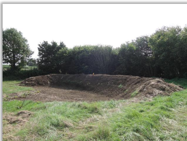
*Bund sited in field corner acting as a sediment trap which was designed to intercept run-off, holding back water and letting sediment settle before reaching the watercourse*
